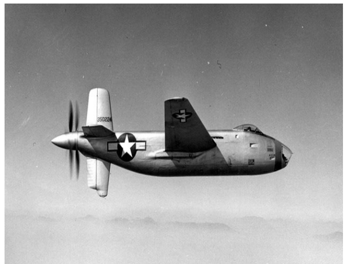
Douglas XB-42 Mixmaster, an experimental bomber aircraft, designed to have a very high top speed (1944).
