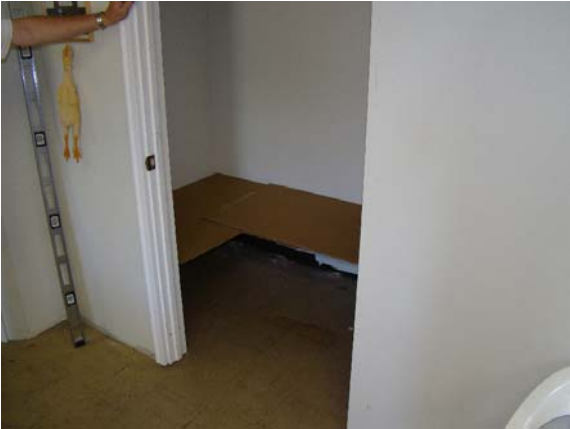
Here's a cardboard template on the first frame, which was used to get the shape right.
