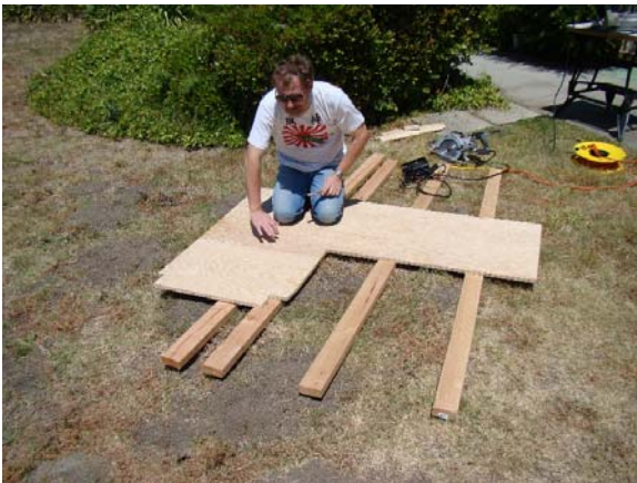
Cutting the plywood to fit.
